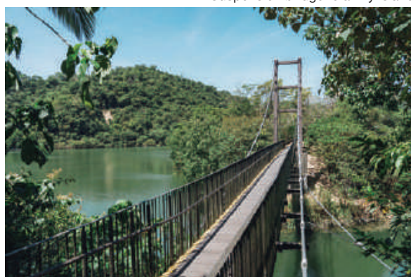
Suspension bridge to a tiny island
